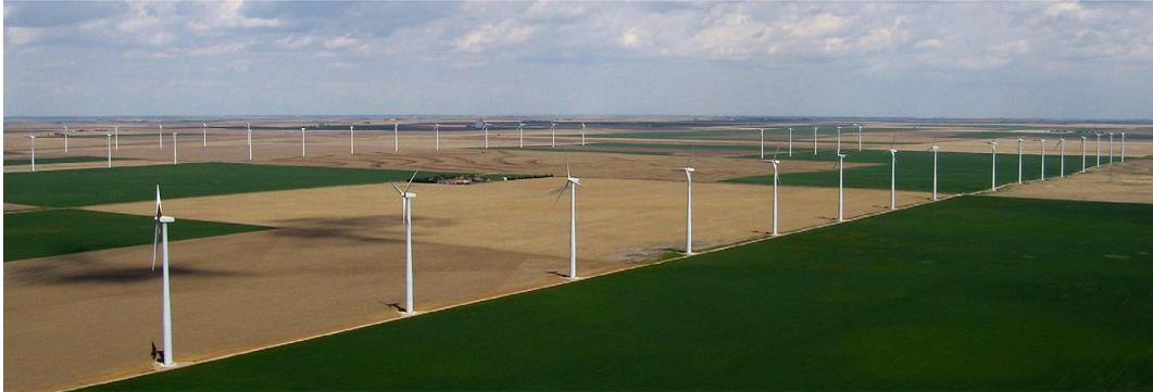
Figure 1. Gray County Wind Farm, the first large array of wind turbines erected in Kansas in 2001. Vestas V47 turbines are relatively small and closely spaced along field boundaries compared with newer and much larger wind turbines. Kite photograph by the authors.
