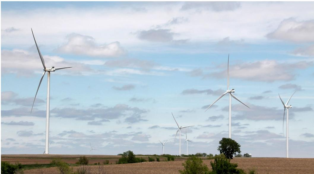
Figure 3. Marshall Wind Energy complex east of Beatite in the glaciated region. Vestas V110, 2.0 MW turbines; towers stand 95 m tall and rotor diameter is 110 m. The turbines are located on a local drainage divide, known as the Summit, between the Roubidoux Creek basin to the west and North Fork Black Vermillion River basin to the east. This wind farm began operation in 2016.
