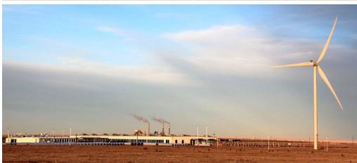
Figure 7. Vestas wind turbines. A – early, small Vestas turbine in operation on the island of Fejø, southeastern Denmark (1987). Note access door and person at bottom of tower for scale. B – Vestas Tower manufacturing plant south of Pueblo, Colorado. V100, 1.8 MW turbine on right was erected in 2010 and is designed for light-wind and/or high-altitude operation.
