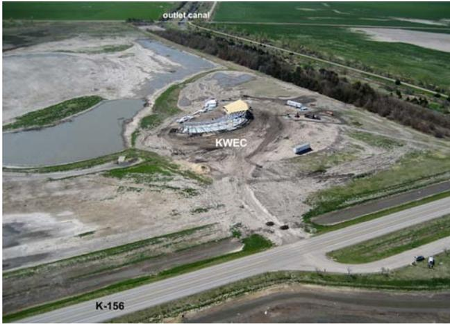
Figure 9. Erecting the Kansas Wetland Education Center next to Kansas highway 156 and the outlet canal for CBWA. Work had to be halted and the foundation raised during flooding of 2007; construction resumed in 2008, when this picture was taken. Note the semi-circular plan of the building and the demonstration marsh behind the building (on left). Kite flyers in lower right corner; May 2008.
