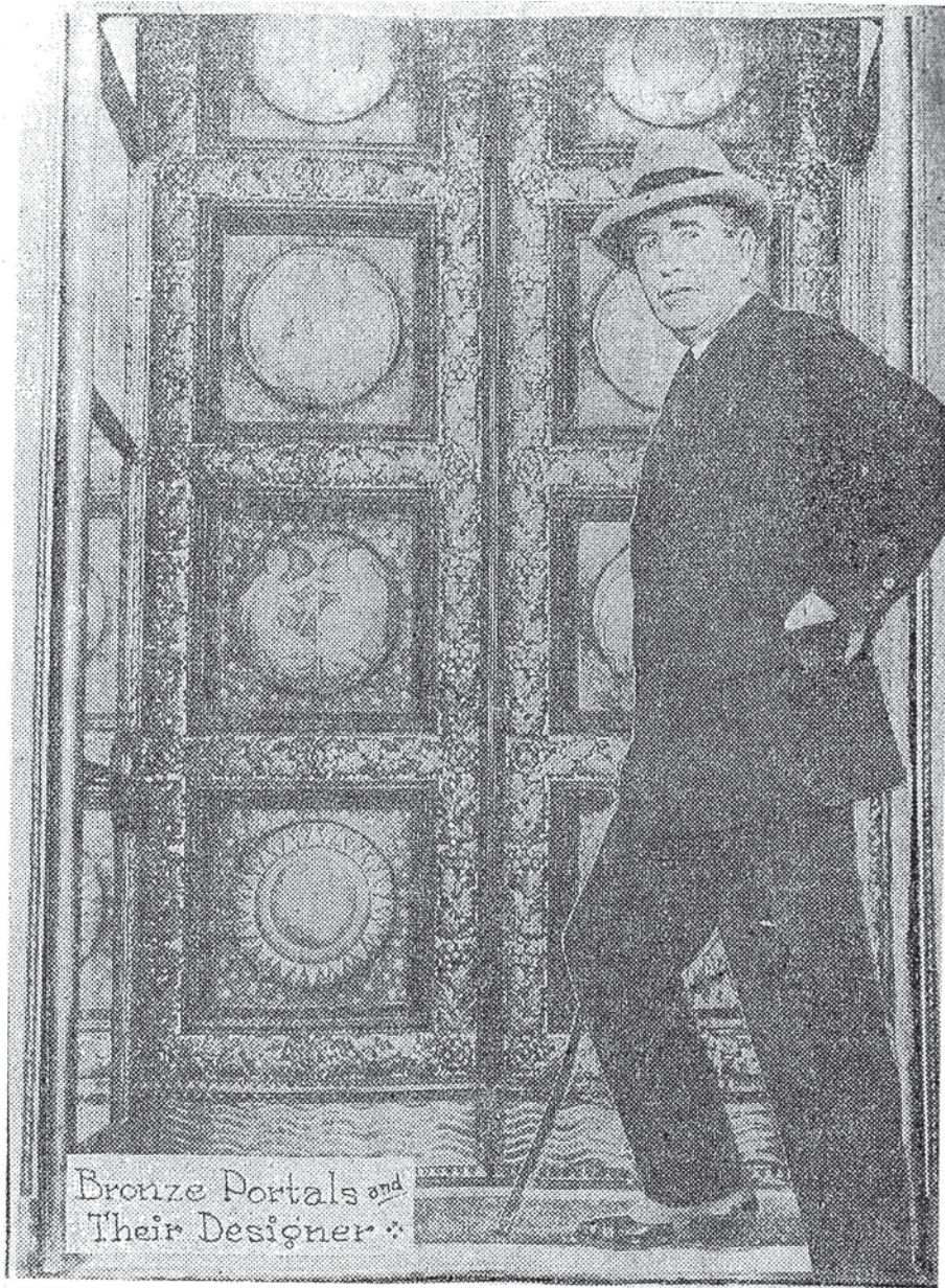
Fig. 27. H. Van Buren Magonigle, Architect of the Liberty Memorial, Kansas City, Missouri. ( Kansas City Star , 7 November 1926).
